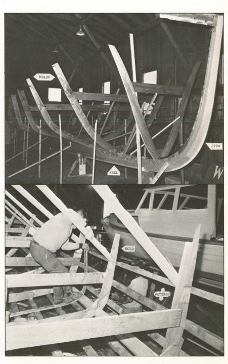
Bert Frost is shown bending in the first steamed oak timber (rib). The molds have been tied together and faired with horizontal battens to which the bent ribs are clamped. Timbering of this thirty-four-foot boat has been completed and the builder, Richard Alley of Beals Island, Jonesport, is planking the hull. He uses cedar plank and Everdur clinch nails. Each plank is shaped, then clamped to the ribs and fastened. The battens are removed one by one as a plank reaches them.
