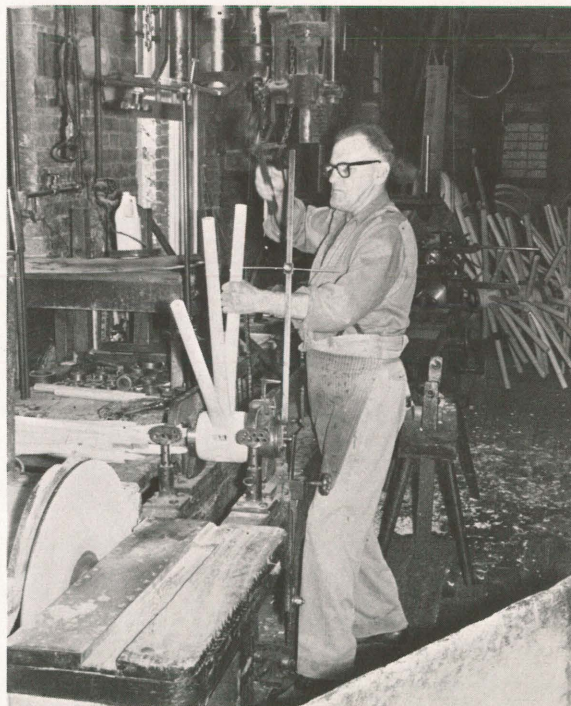
An opportunity to study nineteenth-century machinery and production methods in a vanishing industry was offered industrial archeologists in 1969 when they studied the wooden wheel manufacturing firm of Hoopes Bro. & Darlington at West Chester, Pennsylvania. Shown here is one stage in the manufacture of the wheels produced by the company, most of which are now used for decorative purposes.
