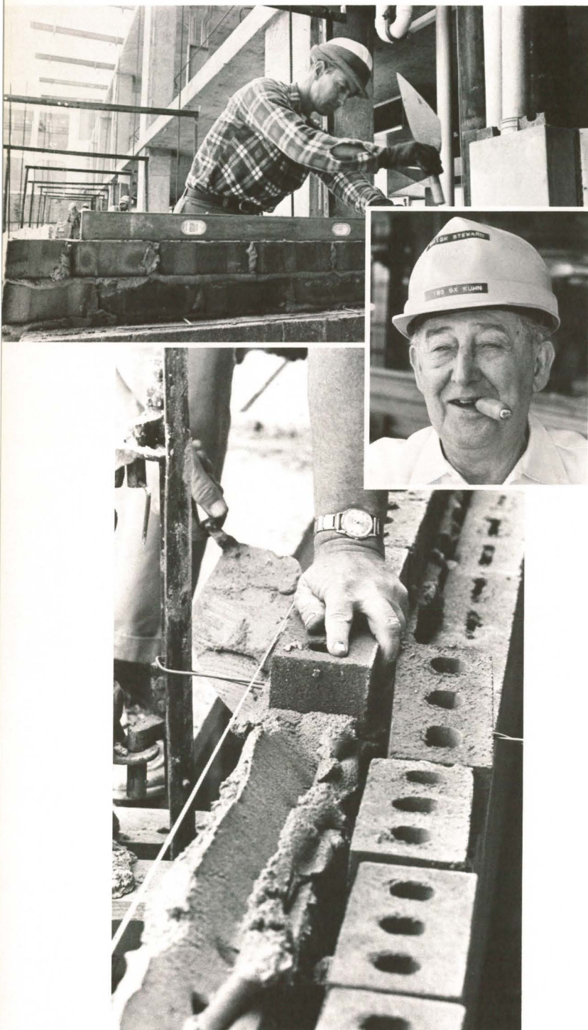
83-year-old Guy Kuhn, a journeyman member, Local 1, of the Bricklayers, Masons & Plasterers since 1911, demonstrates "laying brick to the line" as co-worker "butters the joints." Photo by Lou Hollis
