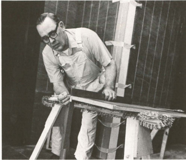
Members of the United Brotherhood of Carpenters and Joiners of America enjoy the challenge of working with solid oak and placing gold leaf trim fitted together in ½" sections like a jig-saw puzzle. Naturally, hard hats are worn on outside construction, but this is finishing off the interior of the Grand Ballroom of the Loew's Hotel, L'Enfant Plaza.
