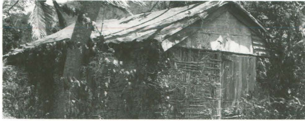
Weathered by years of hurricane seasons, an abandoned wattle and daub house still stands in St. John, its basketwork structure exposed by the elements. (Photo by Fred Nabwooksy)
