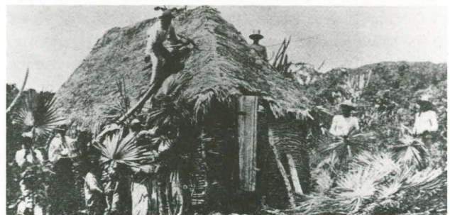
Neighbors construct a thatched roof but in St. Thomas in the 19th century. (Photo courtesy the Virgin Islands Department of Planning and Natural Resources)
