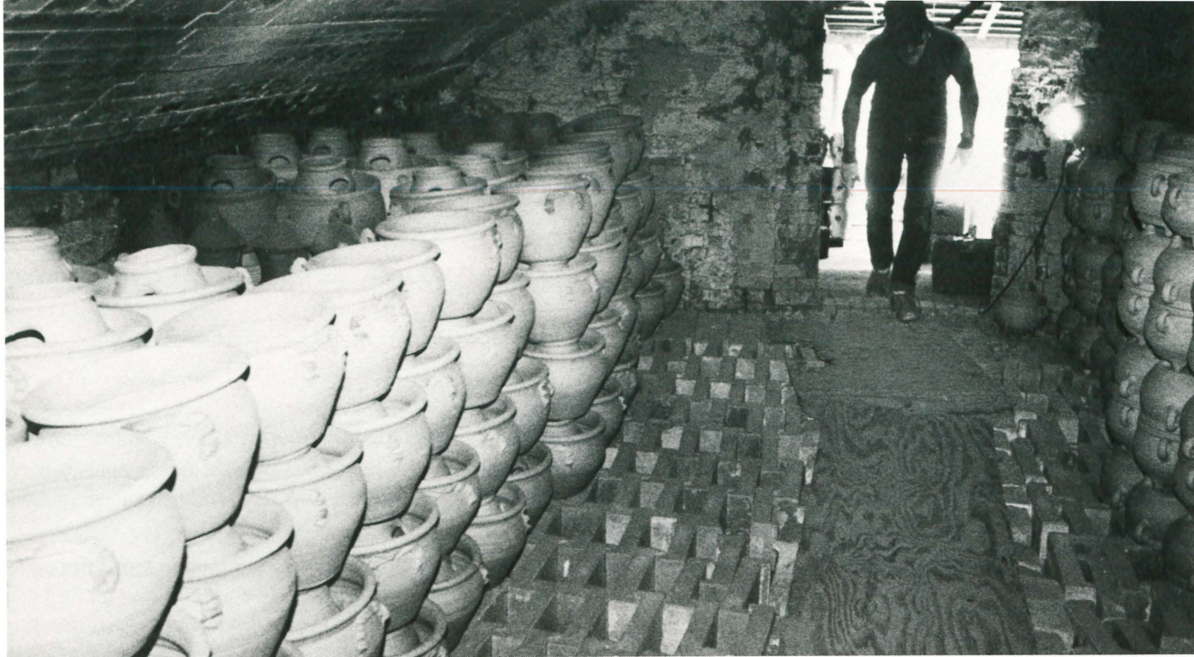
Loading pots in rectangular downdraft kiln. Hewell Pottery, Gillsville, Georgia.
