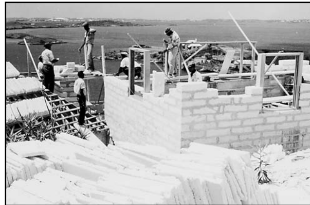
Building using limestone blocks and slate. Courtesy Department of Communication and Information.
